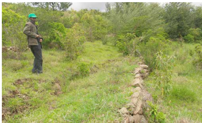
Rehabilitated catchment using excavated trench, stone bunding and grass reseeding at Miriam Monze watershed, Amhara Region
