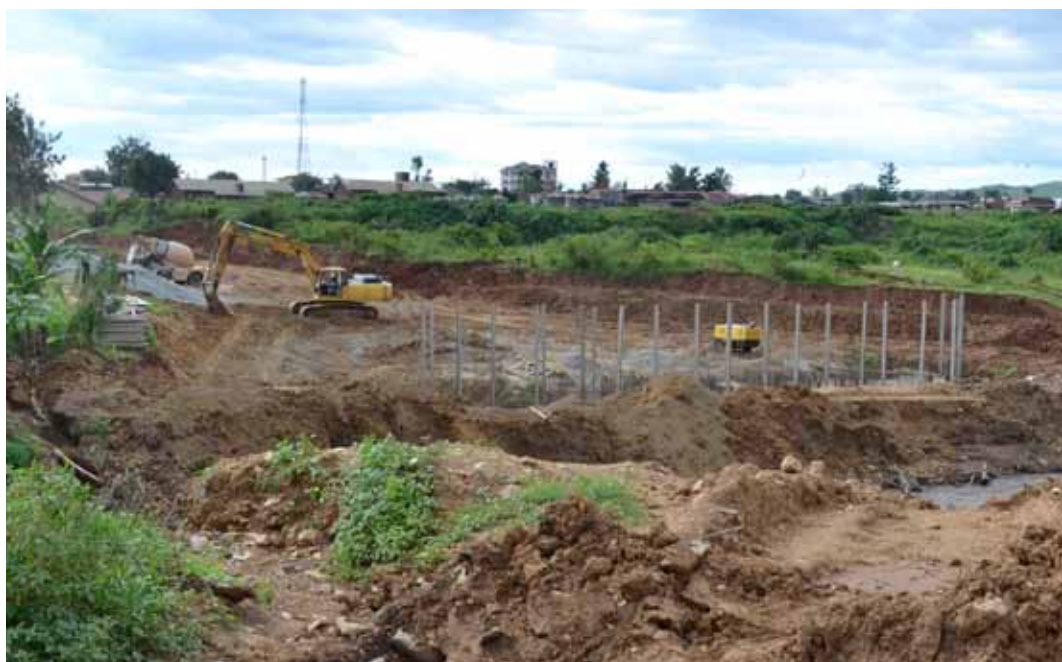
Construction of the Malaba one border post
