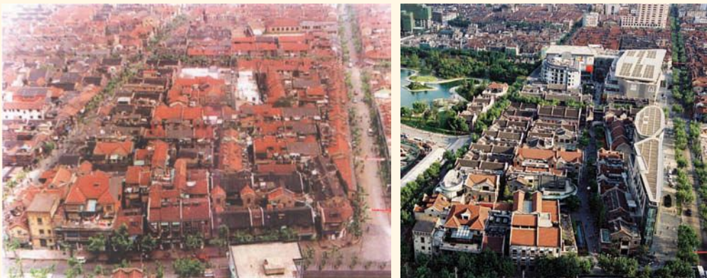
Photograph 6.2 Aerial view of Xintiandi before redevelopment and after redevelopment
